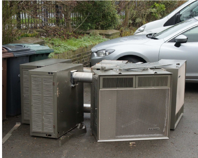
The old gas fired heaters removed
