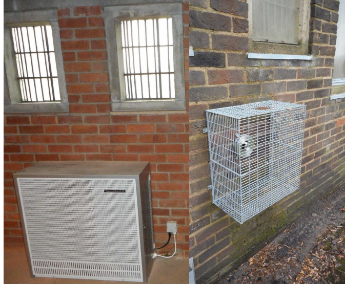
The new completed heater installation
