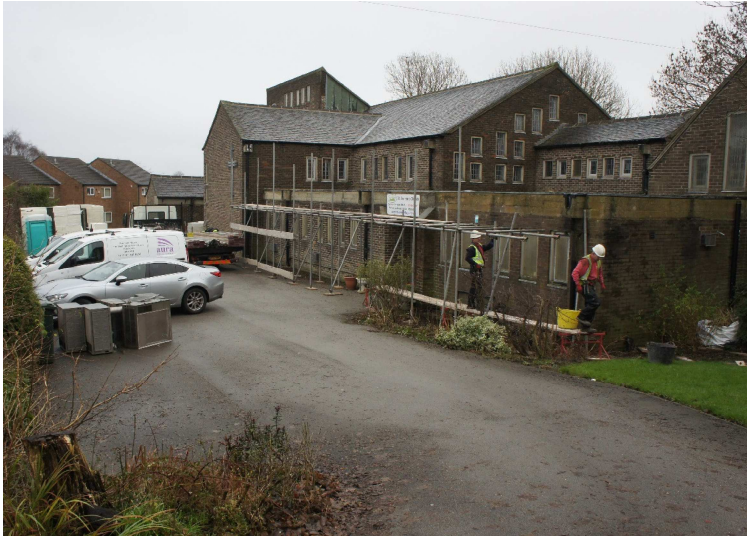
Scaffolding being erected
